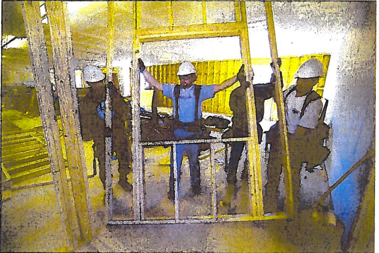
From left, James Bushrod, Vicente Gutierrez, Abel Ortiz and Joel Carabajal add the wall frames last Thursday on the second floor of the Habitat for Humanity of Laramie County Inc. ReStore building at 1804 Ames Ave. in Cheyenne. Hugh Carey/Wyoming Tribune Eagle
